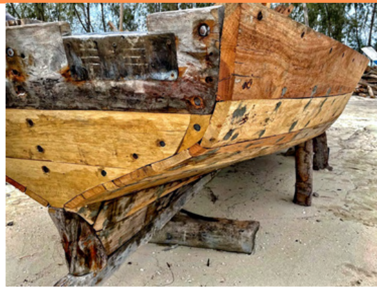
Planking, transom, keel details. Iron spikes are visible. They are wrapped with cotton caulking before they pound them into the planking and counter sink. Later, seam compound and paint is applied to seal.
